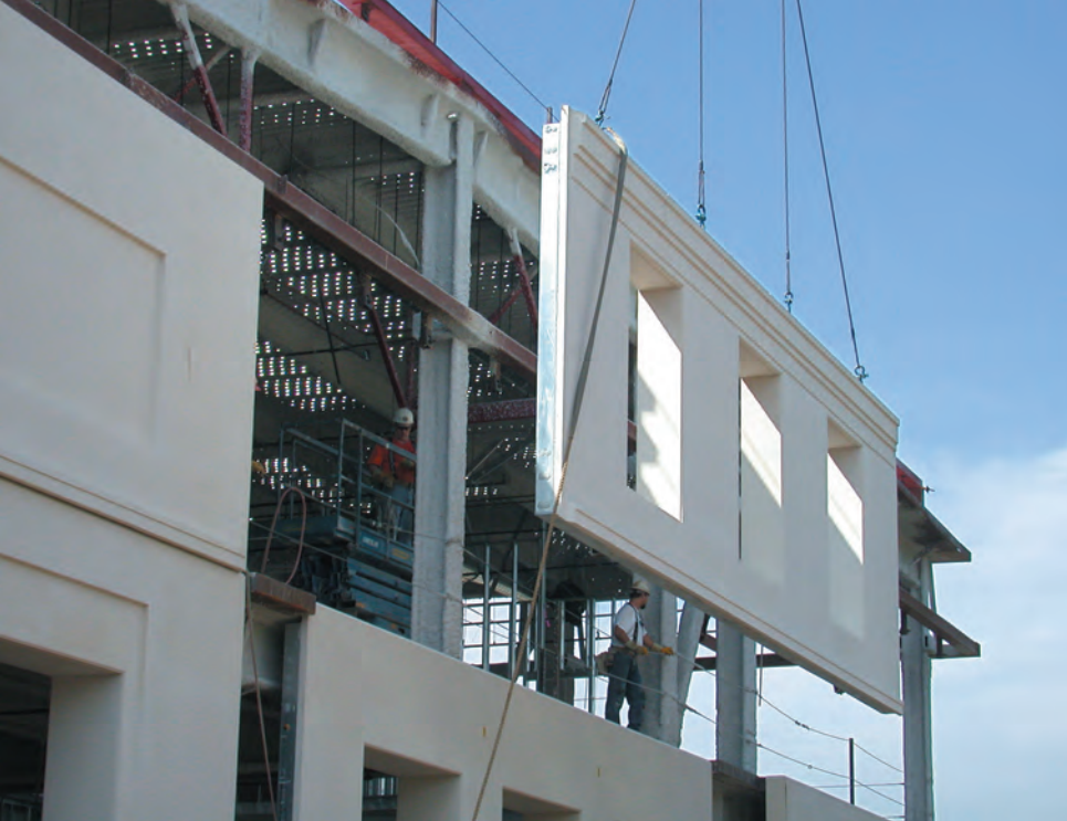
▲ Above: Panels at the Huntington Library had 30-inch-deep returns at windows to create the illusion of massive walls.
